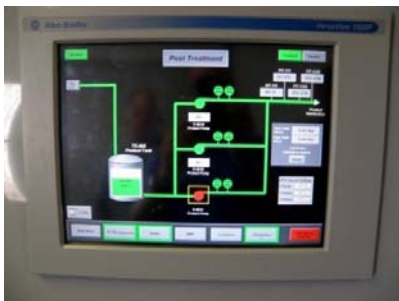
Programmable Logic Computer (PLC) display screen
